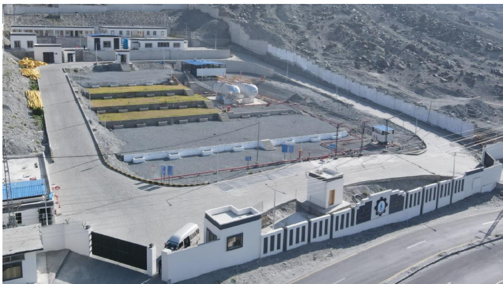
LPG Air Mix Plant- Gilgit
